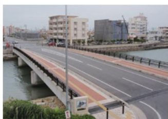
与那原町えびす橋橋梁
